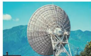
Communication base station
