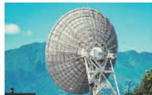
Communication base station
