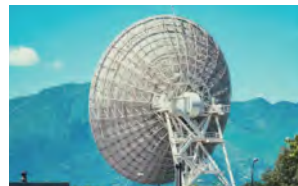
Communication base station
