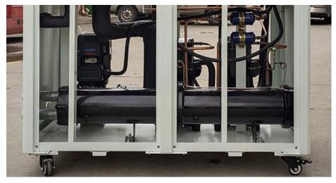
Shell and tube Condenser for water-cooled PET chiller
