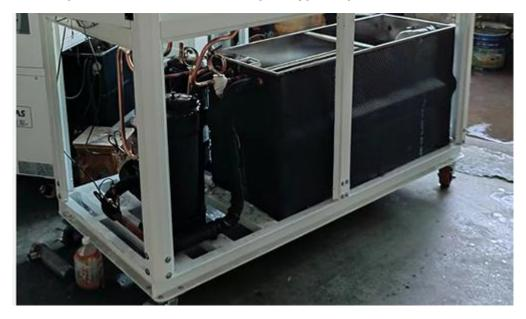
Coil in SS Water Tank Evaporator
