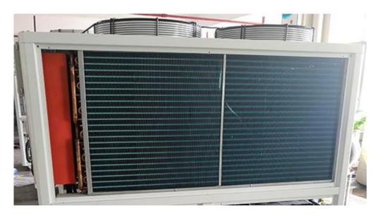
Aluminum fin+fan Condenser for air -cooled MRI chiller
