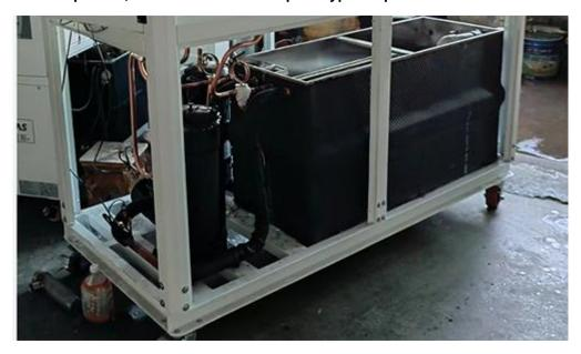
Coil in SS Water Tank Evaporator
