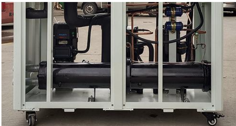
Shell and tube Condenser for water-cooled Extrusion chiller
