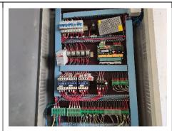
NC #3: Electric box unlocked, no inner cover was installed and electric wires were exposed.
