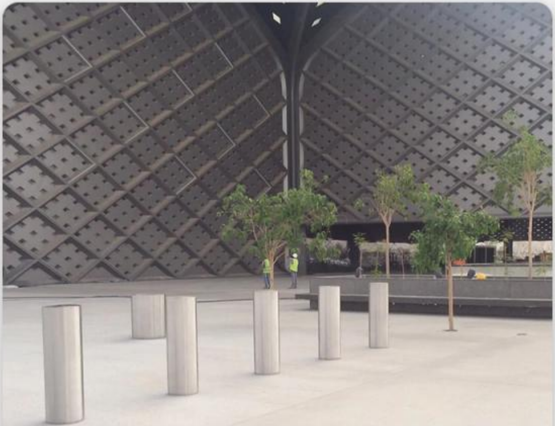
Saudi Arabia Jeddah Railway Station
