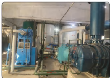
Shandong Sunshine Electric Power
