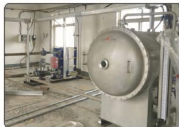
Fujian Rongxin Sewage Treatment Plant
