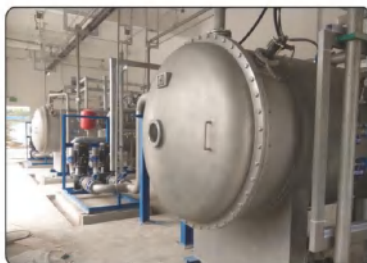
Shandong Binzhou Binbei sewage treatment plant
