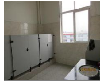
Photo of the sanitary facilities Toilet.JPG
