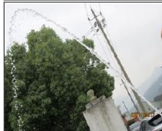
Photo of fire safety equipment 4. Fire hydrant test.JPG
