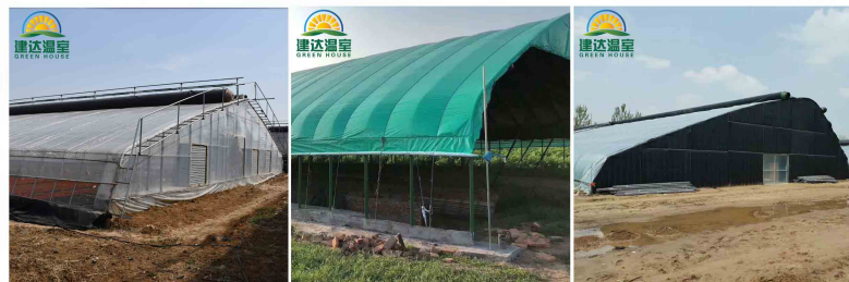
7. LARGE TUNNEL HOUSE
