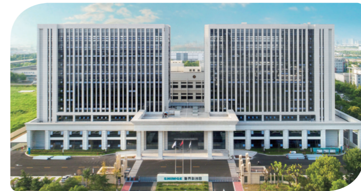
Shime's production base in HangZhou, Zhejiang Province
