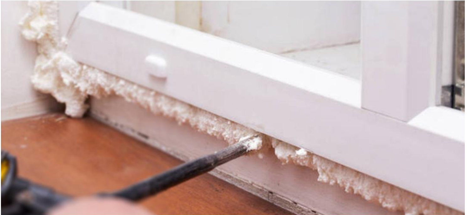
Installation of door and window frames
