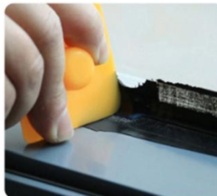
8.Scrape off Any Excess Glue
