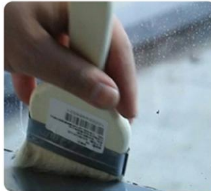
5.Remove Dirt, Grease, Moisture and Old Caulk
