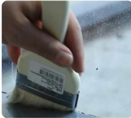
5.Remove Dirt, Grease, Moisture and Old Caulk
