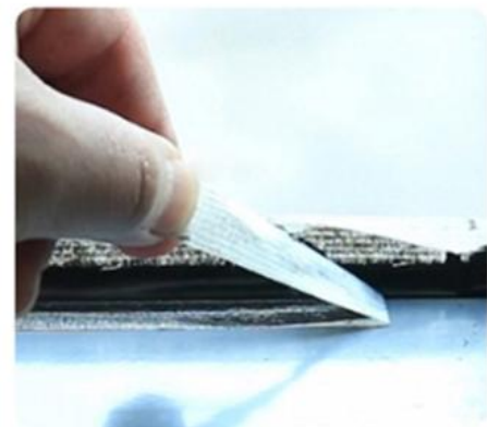
9.Remove Masking Tape Immediately
