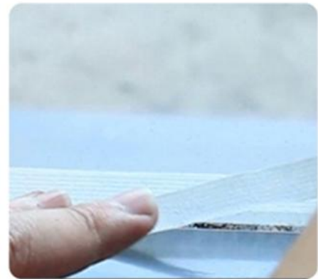
6.Mask Both Sides of Joint With Masking Tape.
