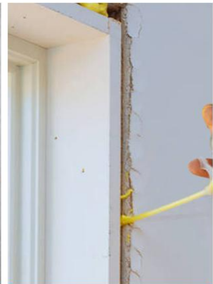
Door and window fixing
