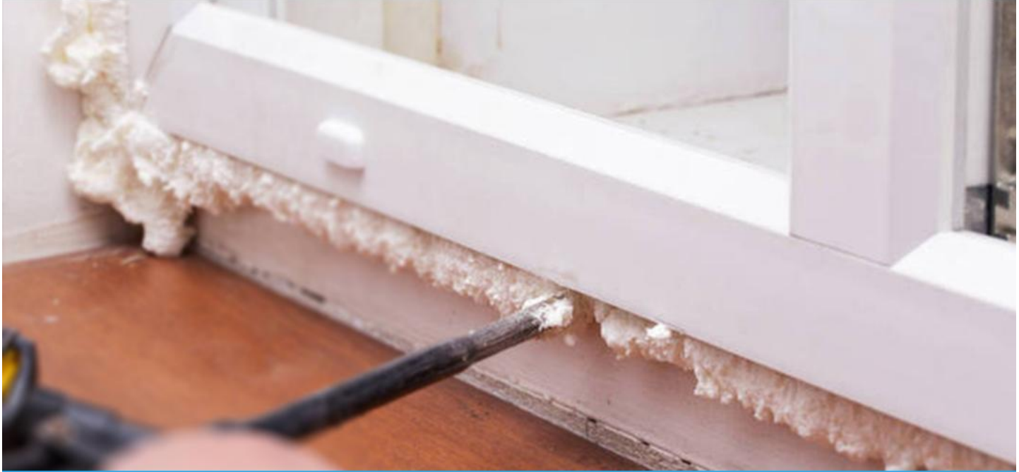
Installation of door and window frames
