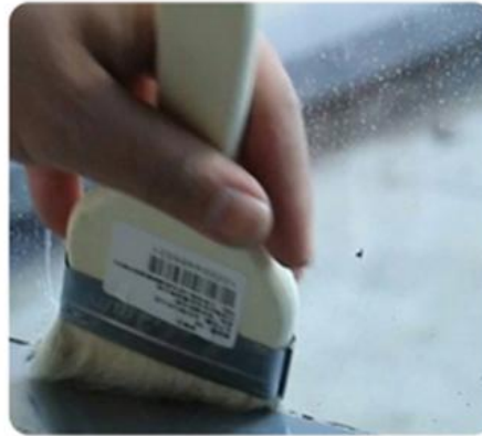
5.Remove Dirt, Grease, Moisture and Old Caulk
