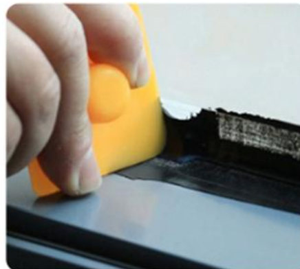
8.Scrape off Any Excess Glue
