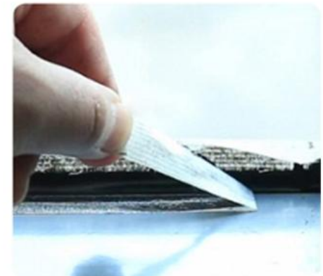
9.Remove Masking Tape Immediately
