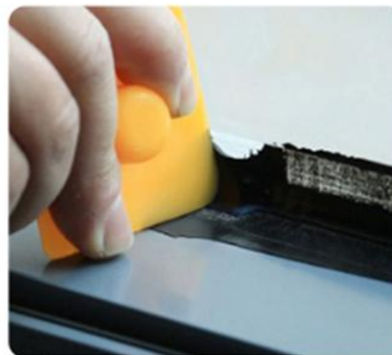
8.Scrape off Any Excess Glue
