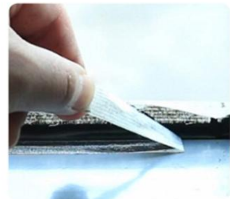
9.Remove Masking Tape Immediately
