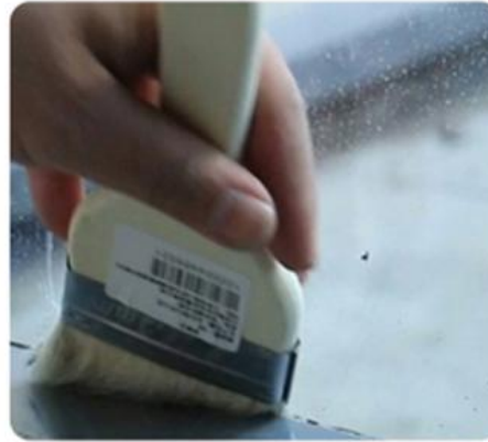
5.Remove Dirt, Grease, Moisture and Old Caulk
