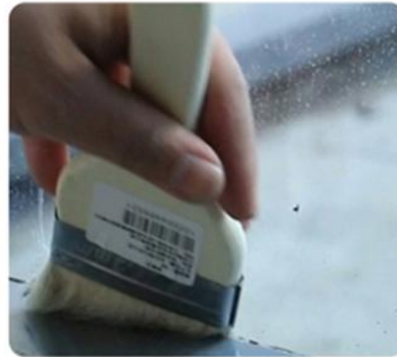
5.Remove Dirt, Grease, Moisture and Old Caulk
