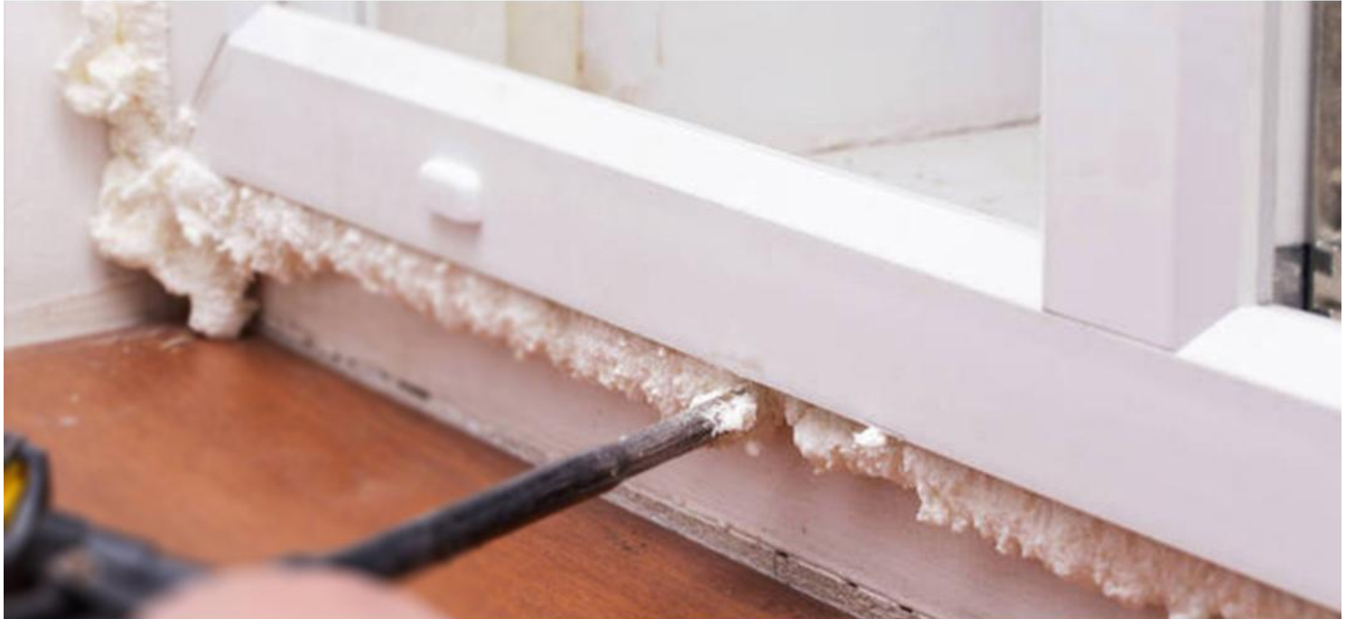
Installation of door and window frames
