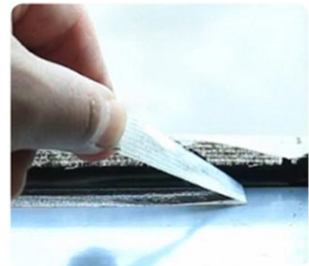
9.Remove Masking Tape Immediately
