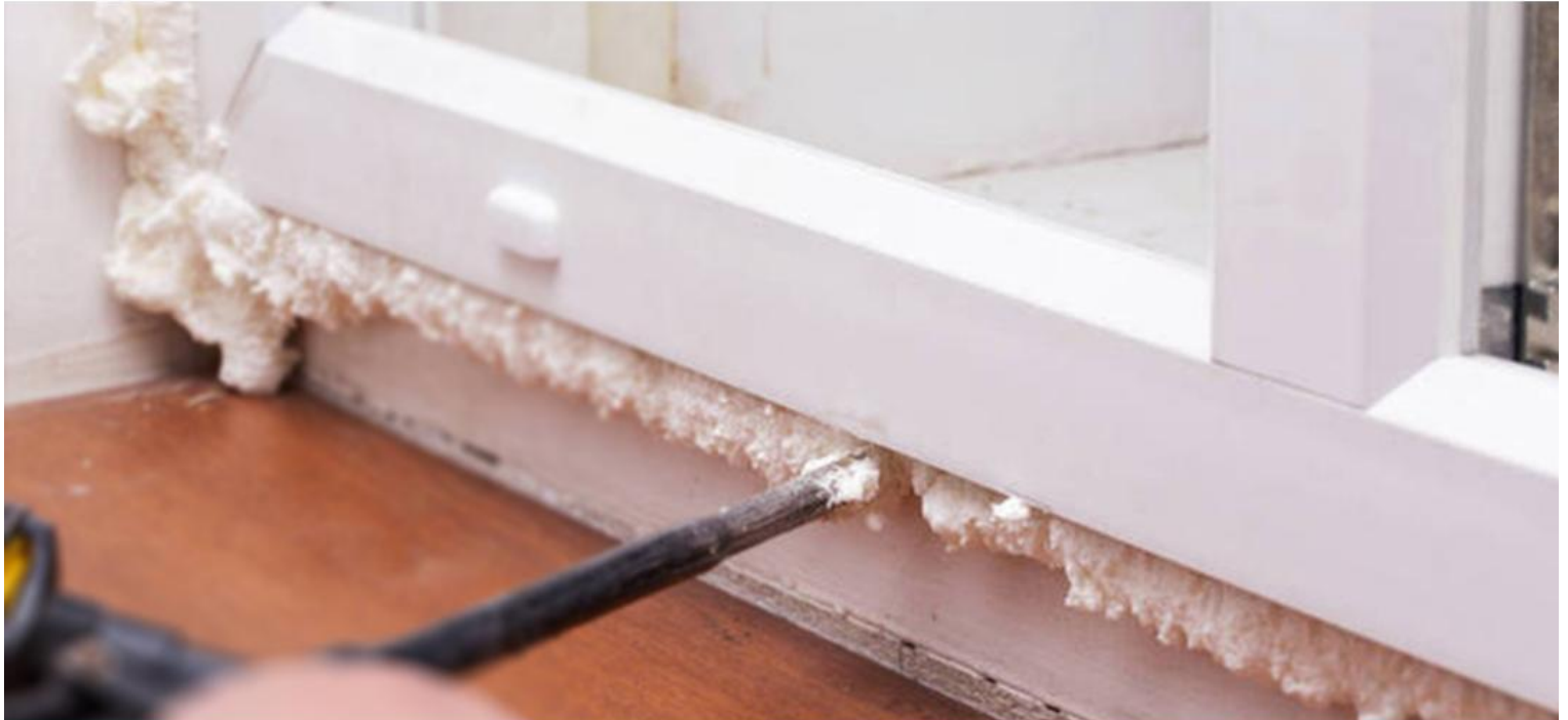
Installation of door and window frames
