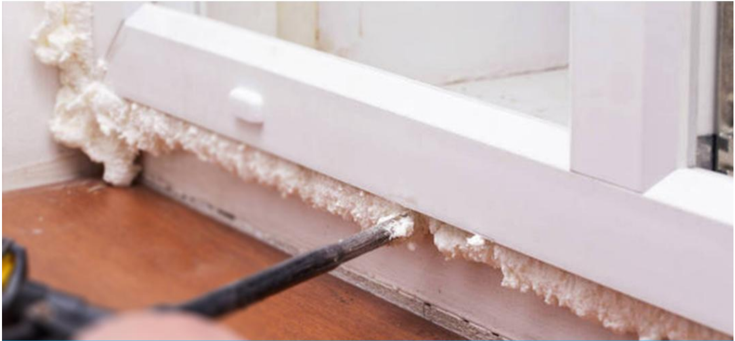
Installation of door and window frames
