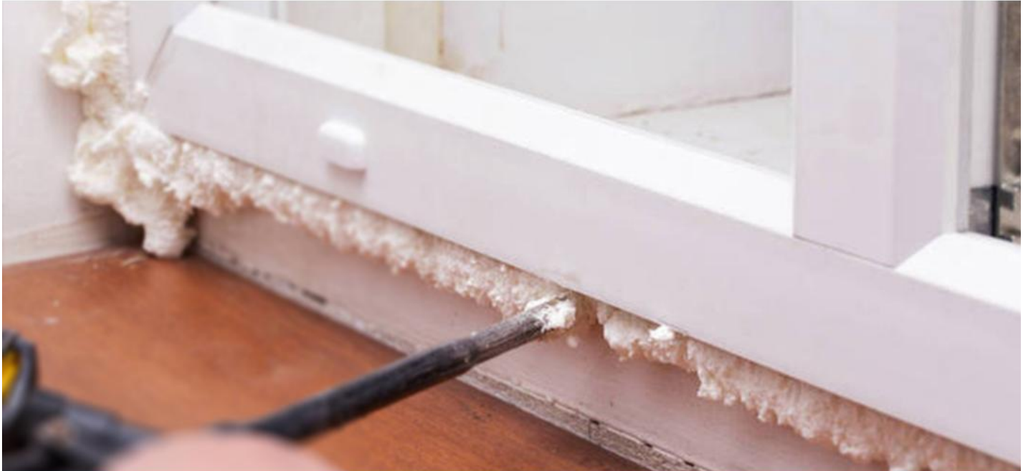
Installation of door and window frames
