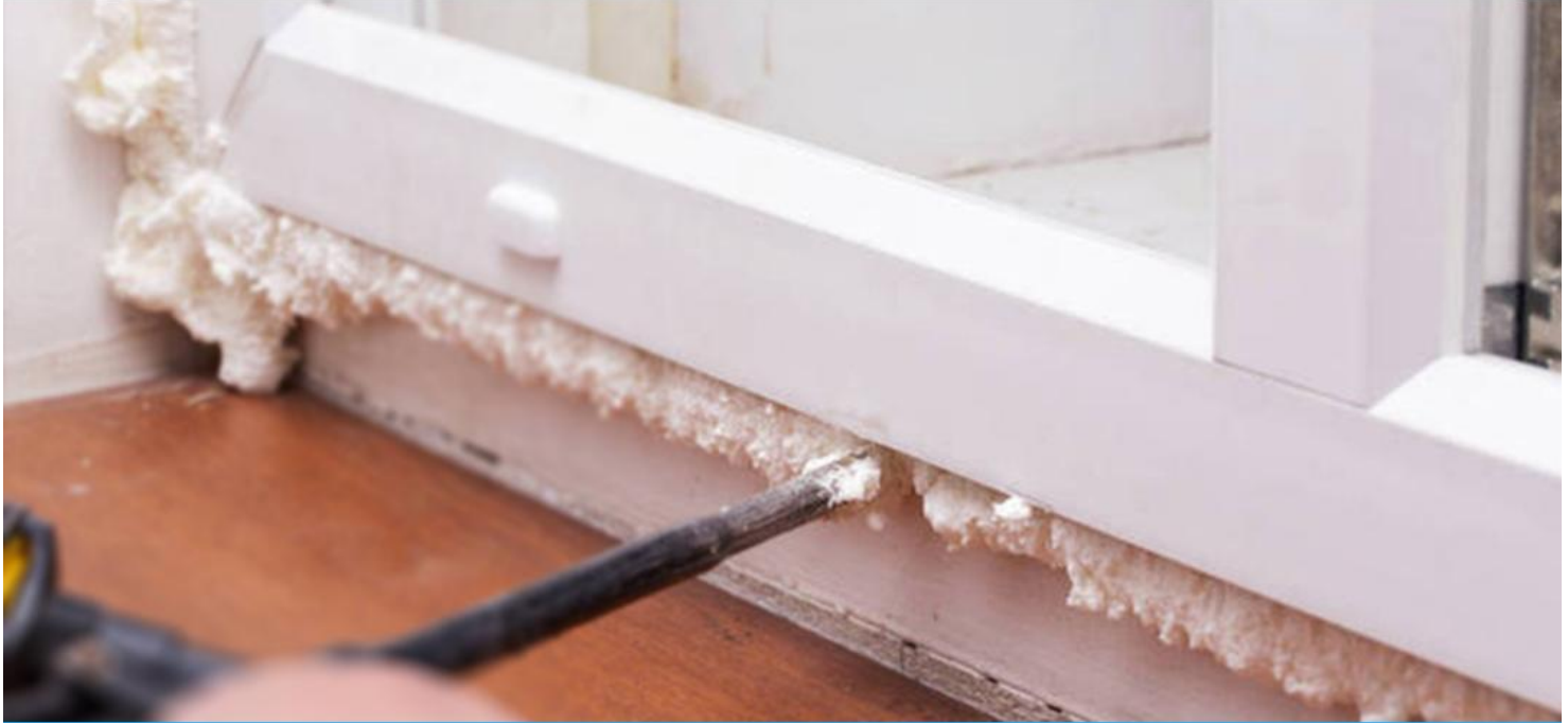
Installation of door and window frames
