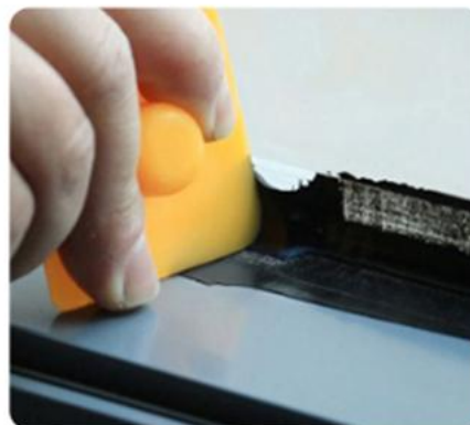
8.Scrape off Any Excess Glue
