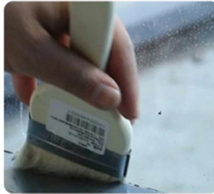
5.Remove Dirt, Grease, Moisture and Old Caulk
