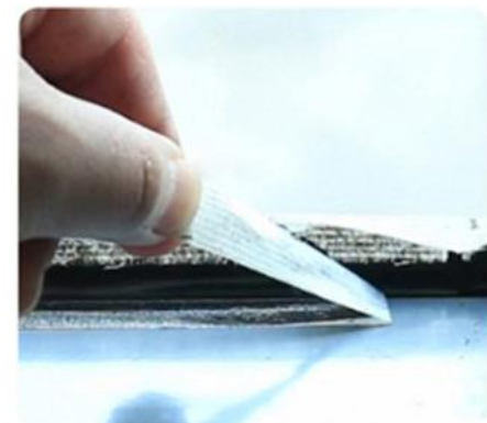
9.Remove Masking Tape Immediately
