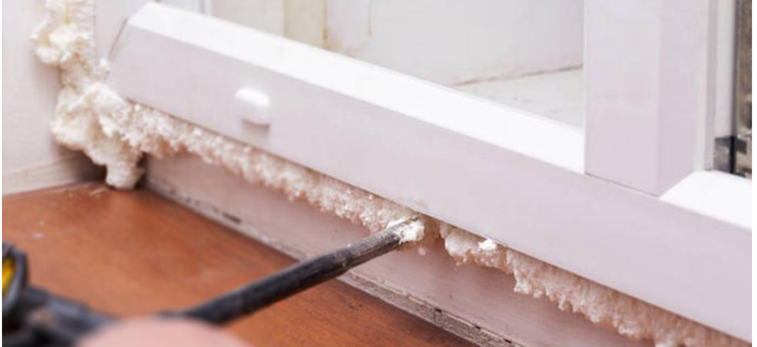
Installation of door and window frames
