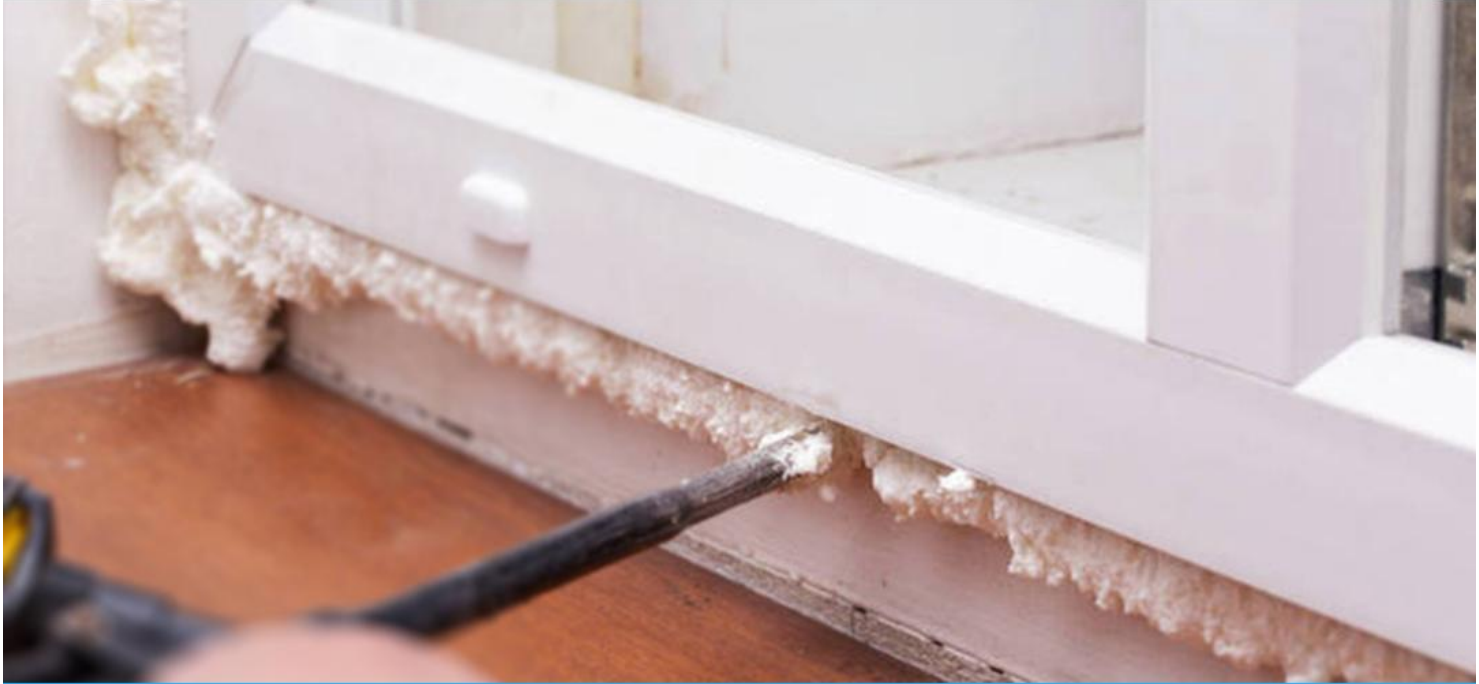
Installation of door and window frames
