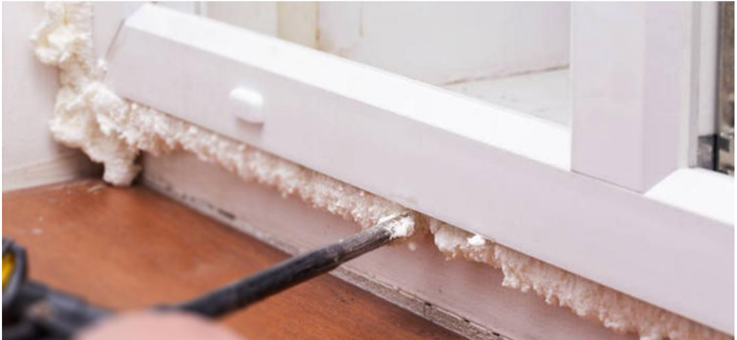
Installation of door and window frames
