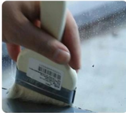
5.Remove Dirt, Grease, Moisture and Old Caulk
