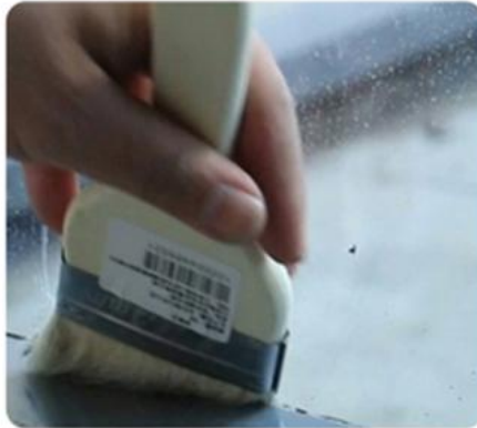
5.Remove Dirt, Grease, Moisture and Old Caulk
