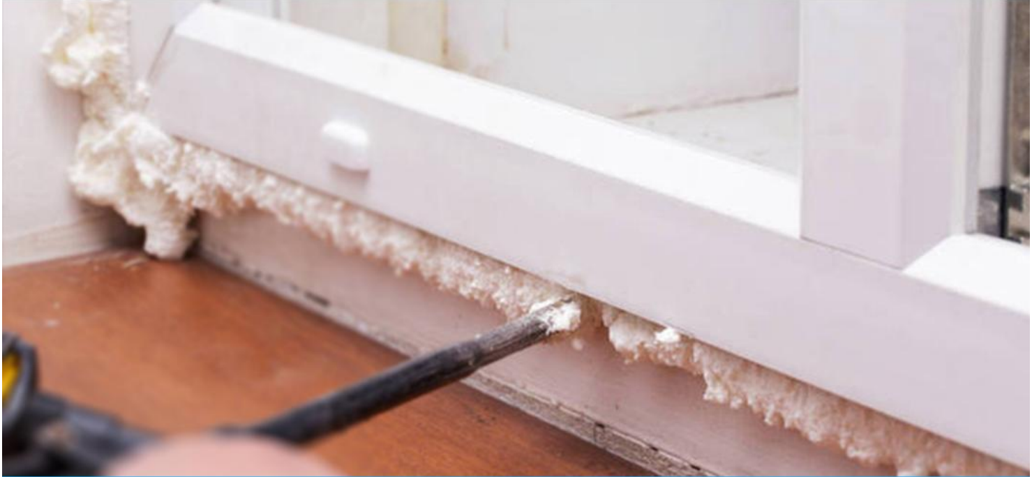
Installation of door and window frames
