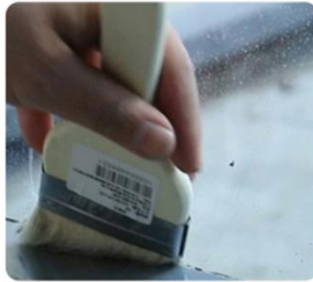
5.Remove Dirt, Grease, Moisture and Old Caulk
