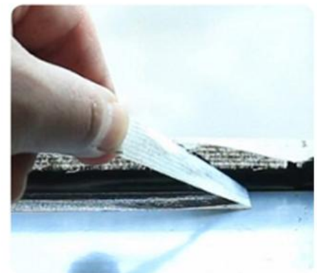
9.Remove Masking Tape Immediately
