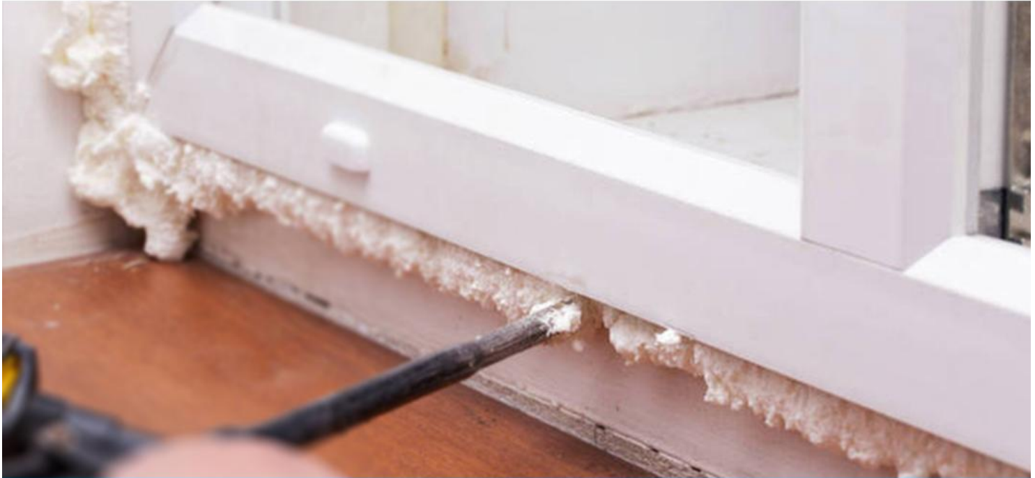
Installation of door and window frames
