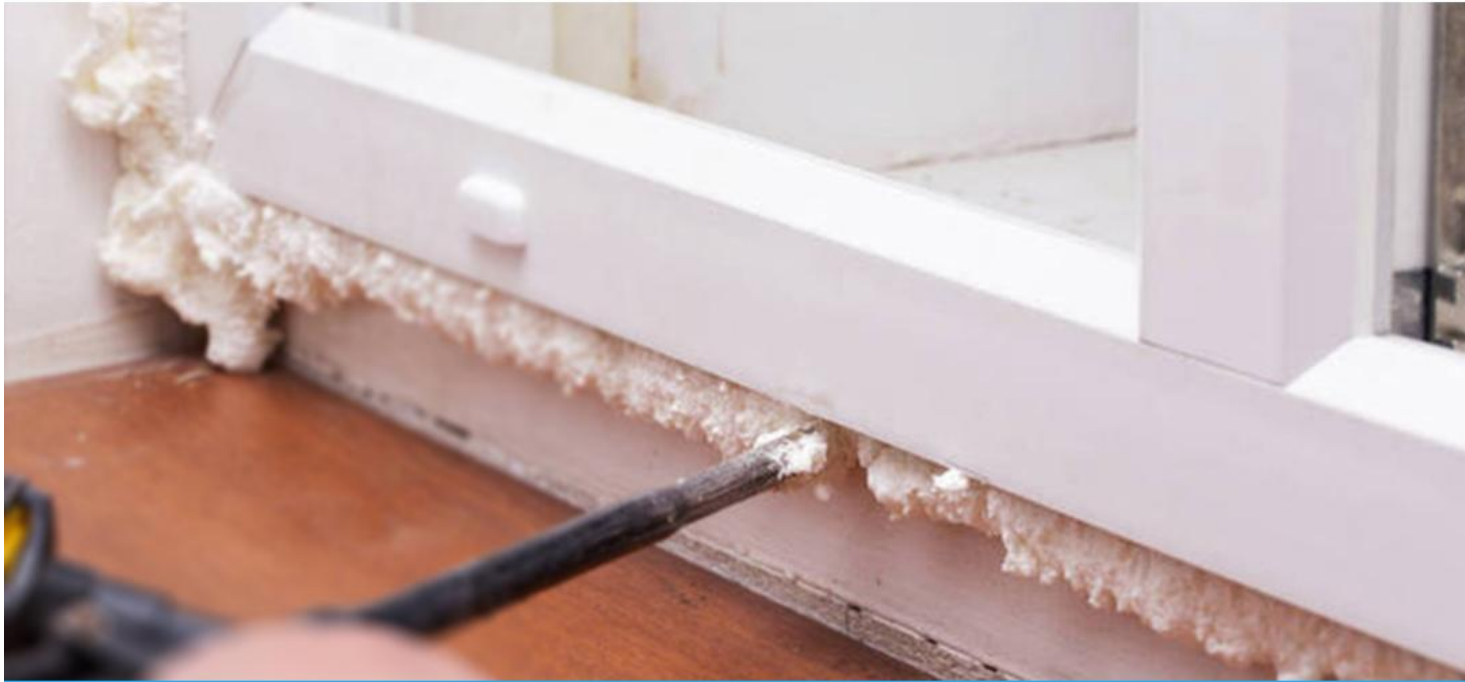
Installation of door and window frames
