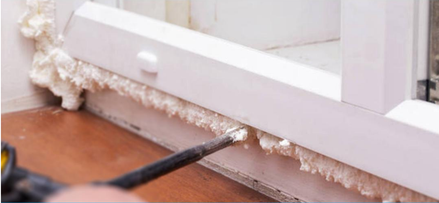
Installation of door and window frames
