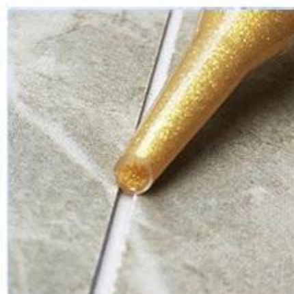
5. Start to fill the sealant into the gap
