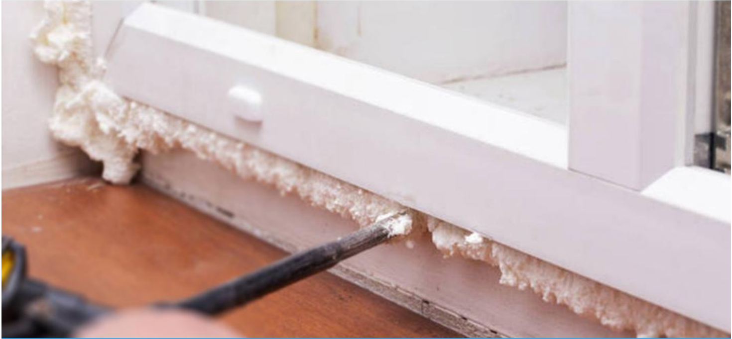
Installation of door and window frames
