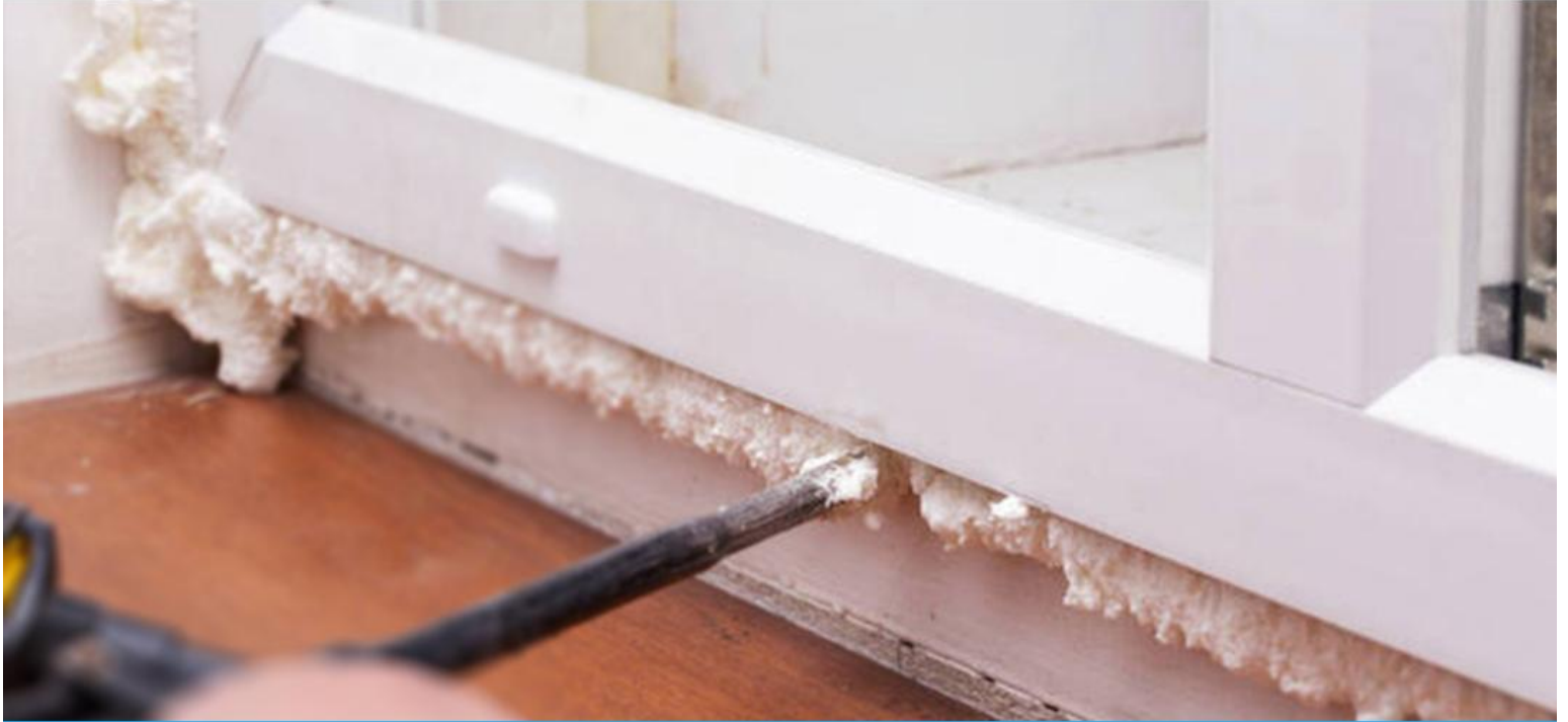
Installation of door and window frames
