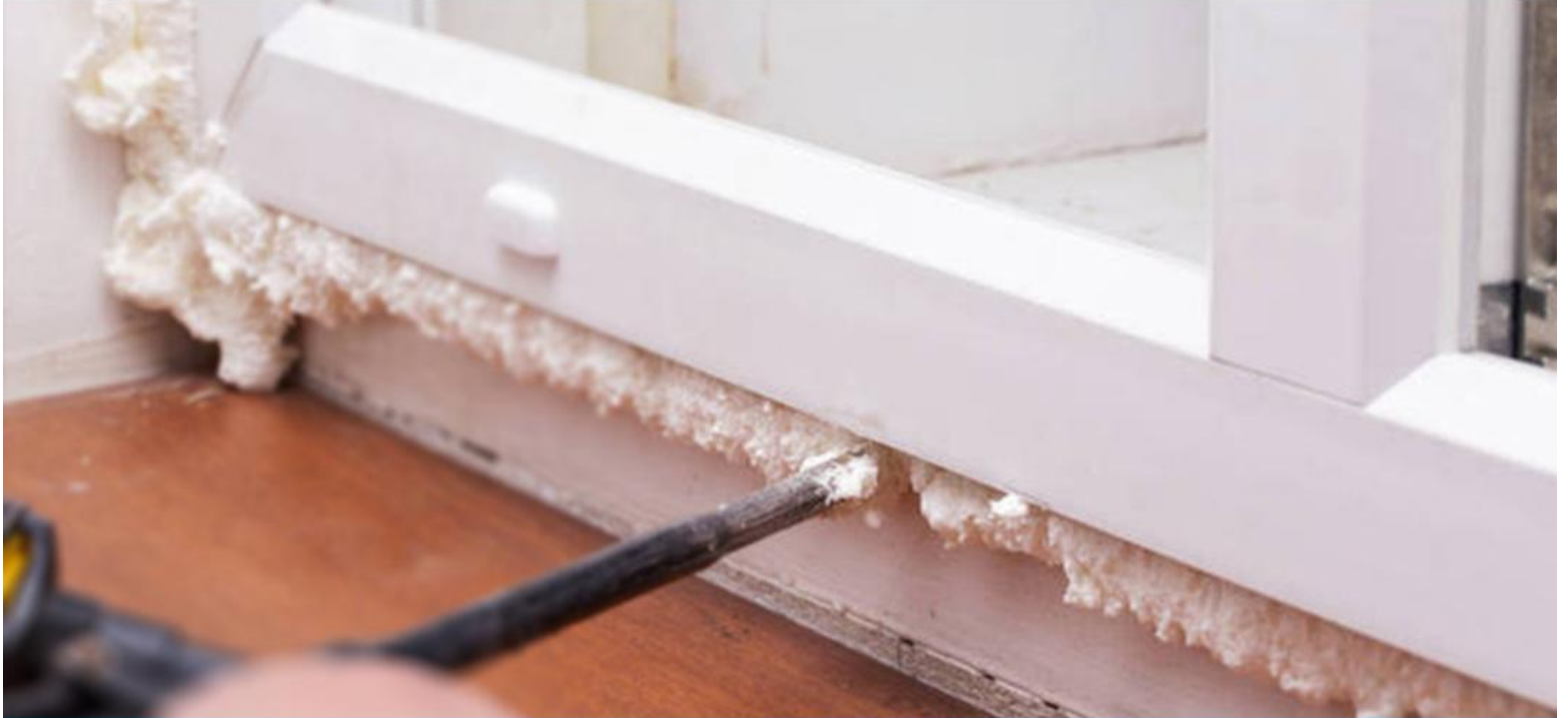
Installation of door and window frames
