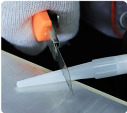
4.Cut Nozzle To Desired Based Size
