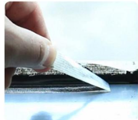
9.Remove Masking Tape Immediately
