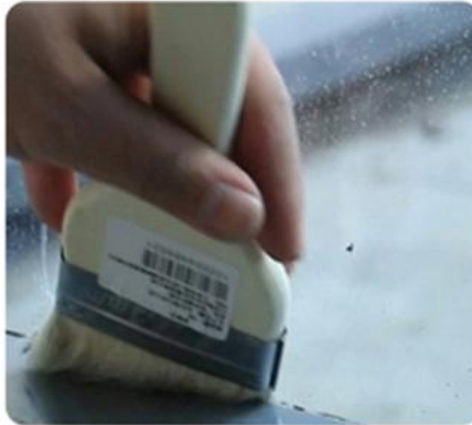
5.Remove Dirt, Grease, Moisture and Old Caulk
