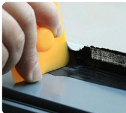
8.Scrape off Any Excess Glue
