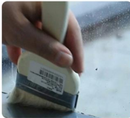
5.Remove Dirt, Grease, Moisture and Old Caulk
