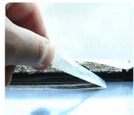
9.Remove Masking Tape Immediately
