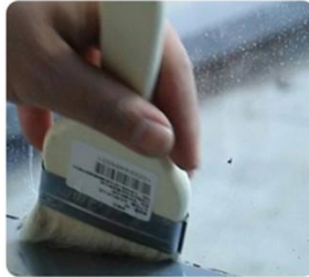
5.Remove Dirt, Grease, Moisture and Old Caulk
