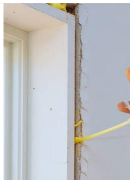
Door and window fixing
