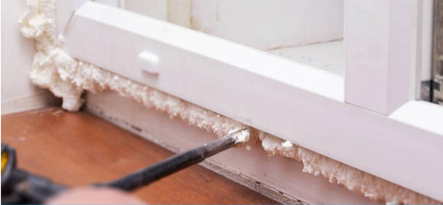
Installation of door and window frames
