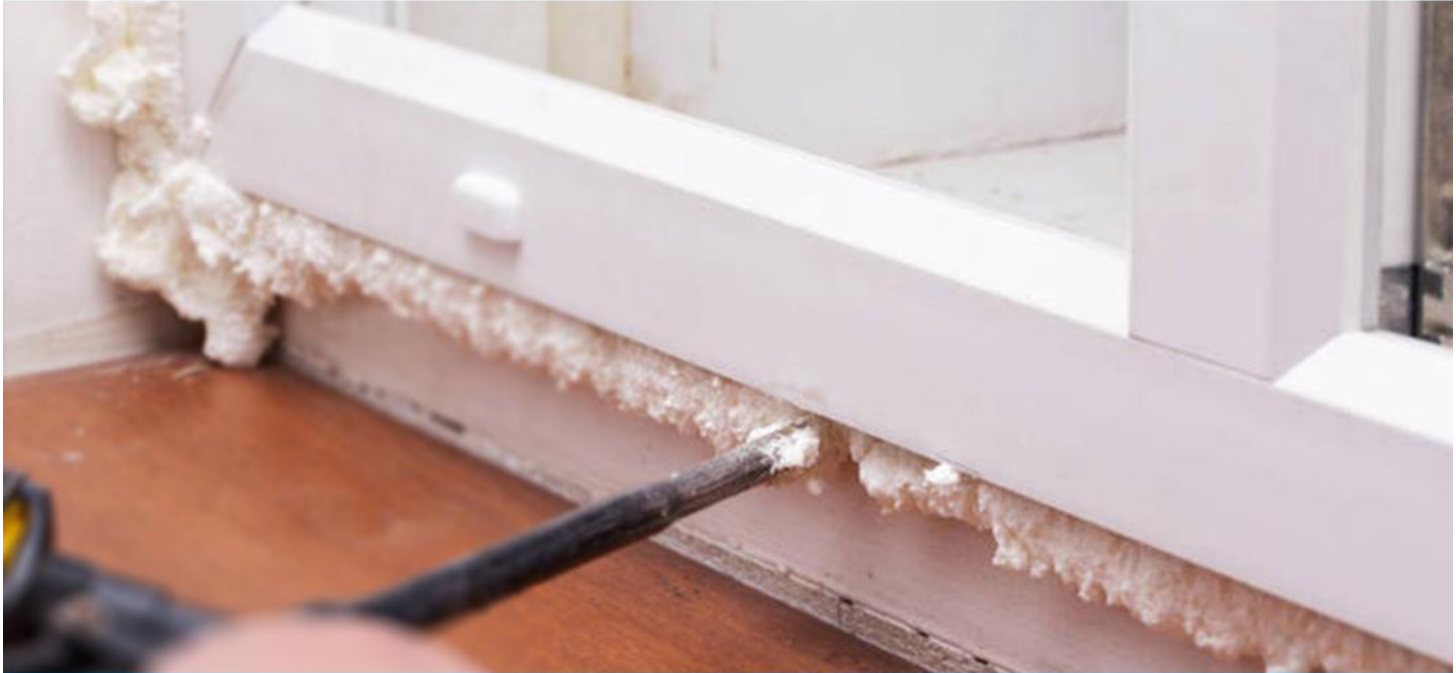
Installation of door and window frames
