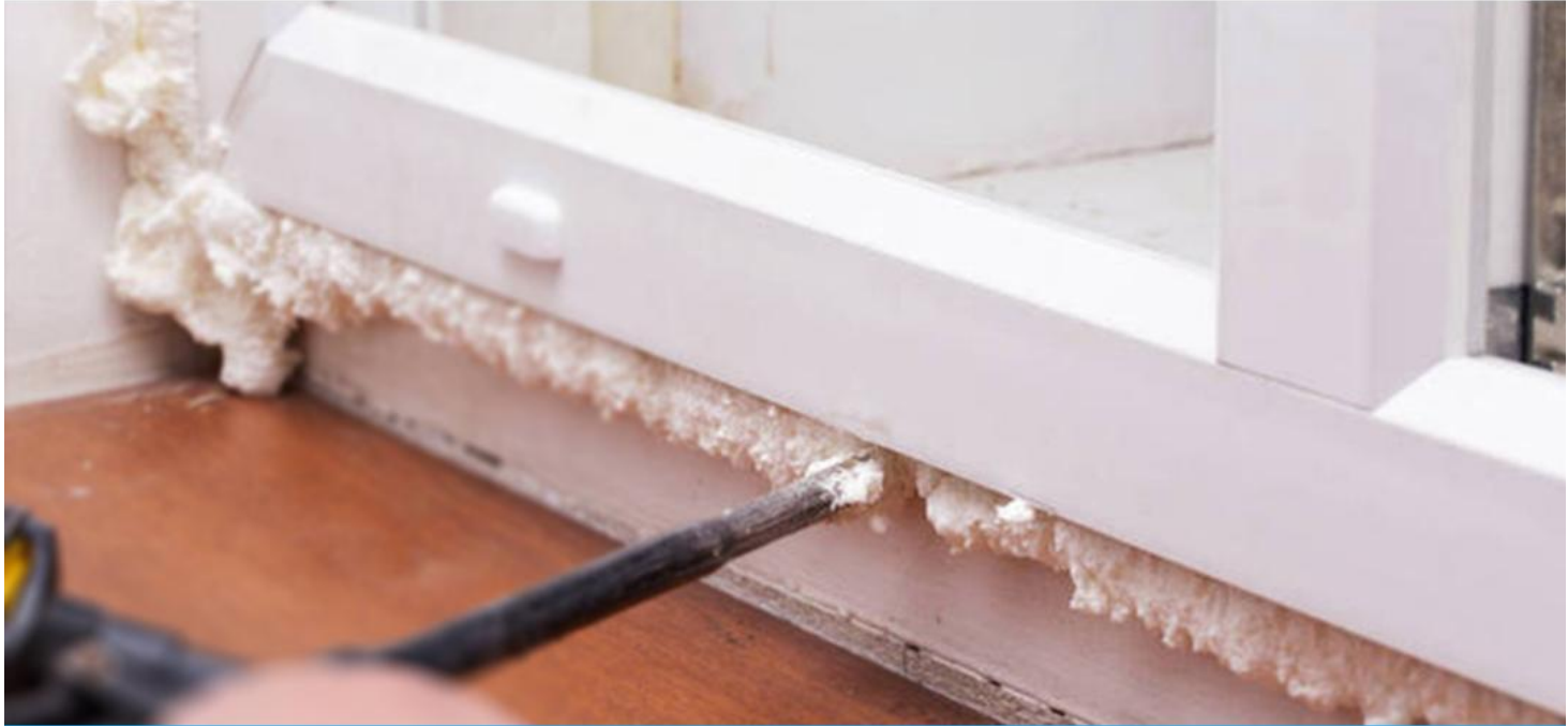
Installation of door and window frames
