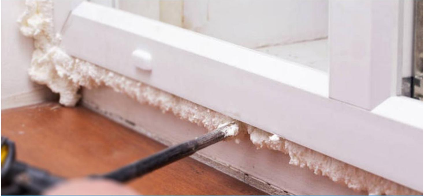
Installation of door and window frames
